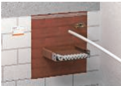
Simple retroinstallation through removal or cutting of individual blocks
