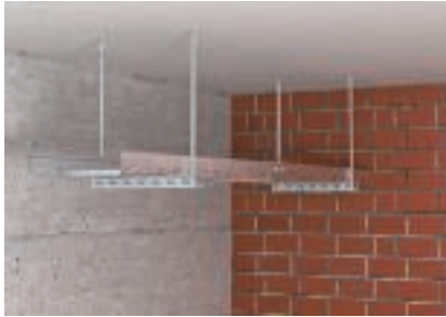
Single-layer ceiling suspension
