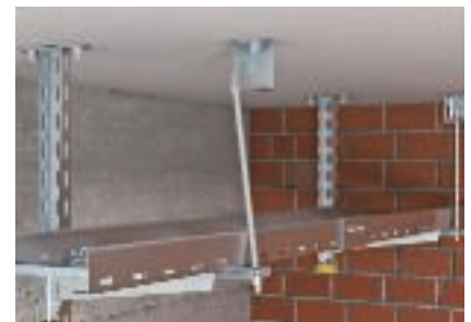
Attachment of the threaded rod in the fire protection clamp
