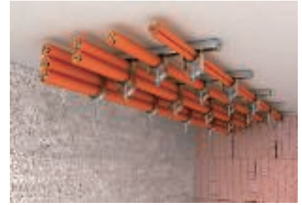
Horizontal cable mounting with clamp clips under the ceiling
