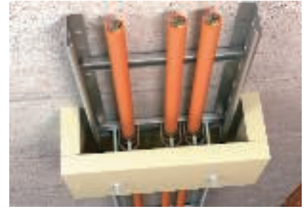
Mounting of the strain relief in combination with vertical ladders
