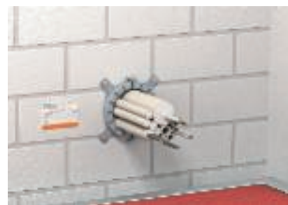
Labelled insulation of installation pipe bundles
