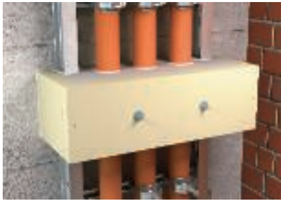
Effective support measure with ZSE90 strain relief
