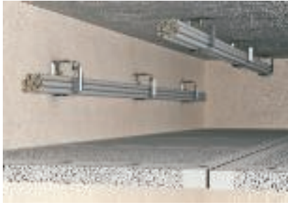
Wall and ceiling mounting above suspended fire protection ceiling
