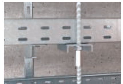
Threaded rod fastening on the tray with multi-layer arrangement
