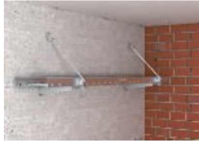
Wall mounting with diagonal threaded rod locking
