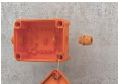
Cable entry with V-TEC cable glands
