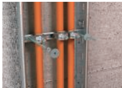
Fastening with threaded rods and slide nuts in the rungs
