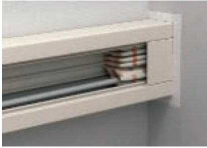
Cushions arranged in the duct
