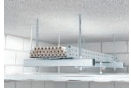
Required minimum spacing to the fire protection ceiling
