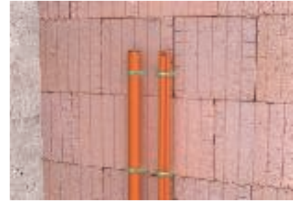
Vertical cable installation as individual and bundle routing on the wall
