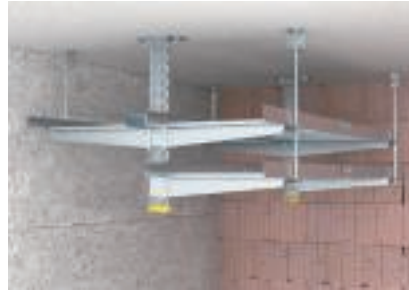
Ceiling mounting with bracket arrangement on both sides
