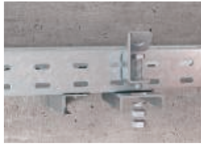
Fastening of the sloping connection component
