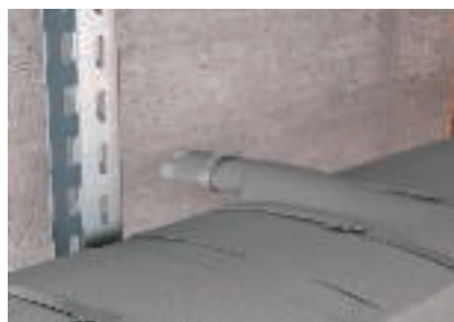
Cable exit with bandaging
