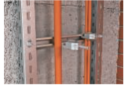
Installation of the cables with clamp clips, also possible in the case of multiple assignment
