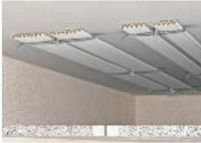
Ceiling mounting above suspended fire protection ceiling
