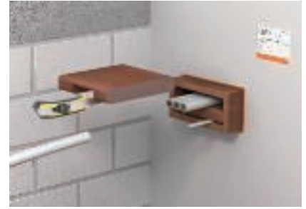
Exact cutting of the internal pieces and then insertion in the frame
