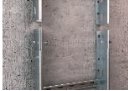
Joint connection with screwed-on connector
