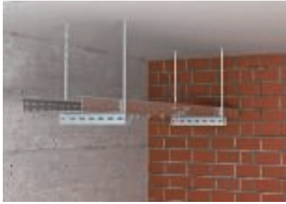
Single-layer ceiling suspension
