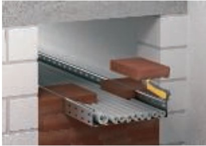
Mounting of the cut blocks
