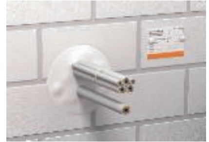
Labelling of the small insulation
