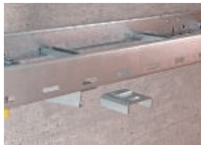
Attachment of the connection component on the underbelt of the ladder rail
