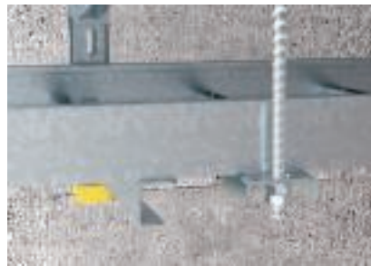
Connection component at a spacing of max. 100 mm next to the bracket
