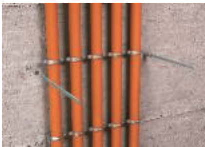
Fastening points next to the cables directly on the wall
