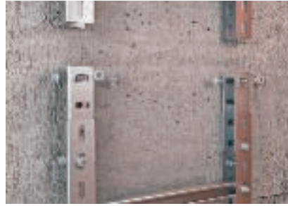
Joint design with screwed-on connector
