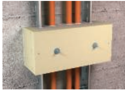
Effective support measure with ZSE90 strain relief
