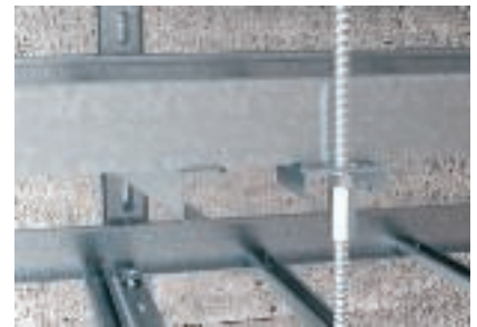
Threaded rod mounting for multi-layer route arrangement
