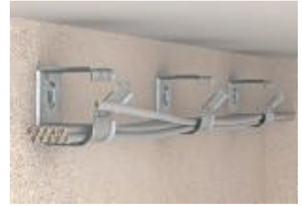
Simple insertion the cables in the opened grouped support
