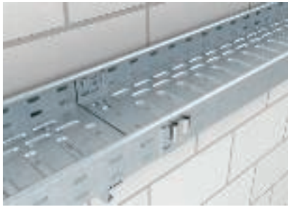
Connected joint connector, only the base shackles need to be bent
