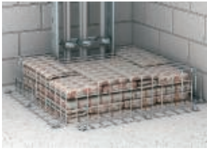
Lock against slippage above the floor
