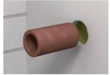
Insertion of the pipe shell in the light-duty partition
