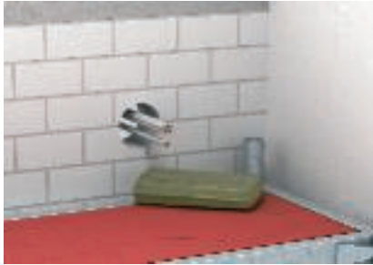
Mineral wool with melting point \geq 1,000 °C to plug the opening
