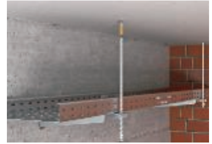
Ceiling fastening of the threaded rods with internal thread clamps
