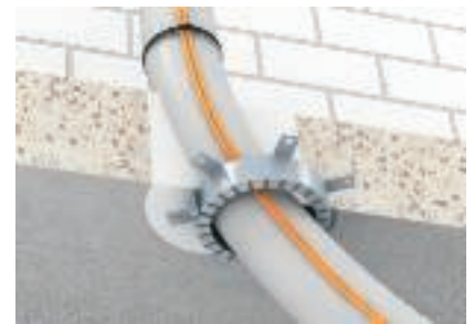
Pipe post systems with 2 accompanying cables
