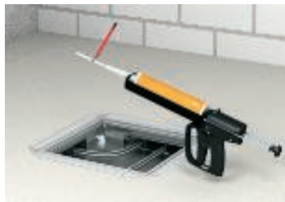
Use of the mixing tube with extension to apply the fire protection foam
