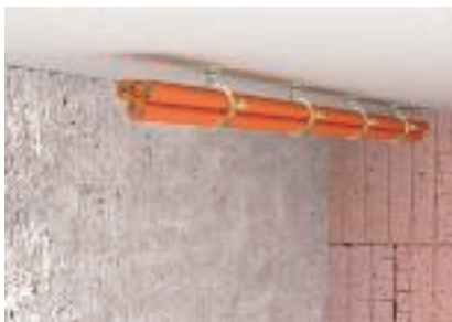
Bundled cable routing under the ceiling
