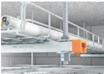
Clamp fastening for high load capacities
