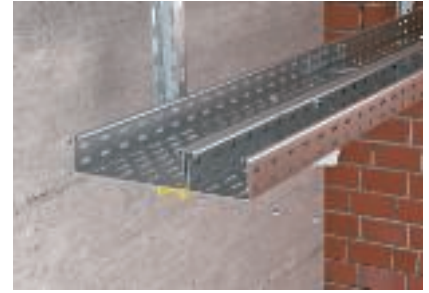
Mounting of two cable trays jointly on one bracket
