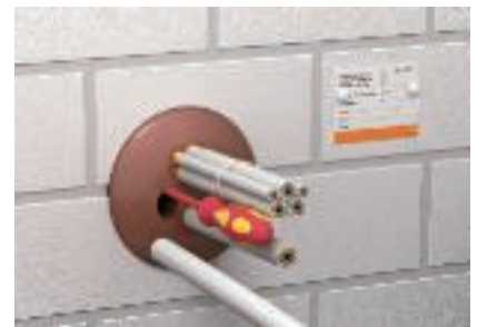
With retroinstallations, careful cutting and drilling of the plugs
