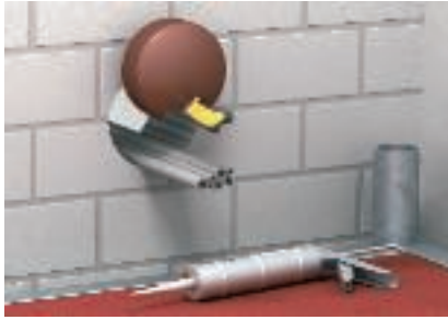
Cutting of the plugs for cable assignment on the edge of the core hole
