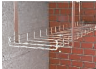
Fastening of the mesh cable tray with clamping piece and truss-head bolts
