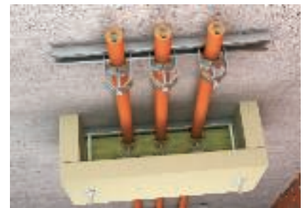
Effective support measure with ZSE90 strain relief
