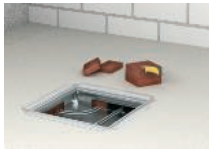
Cutting of thin strips for the duct compartments
