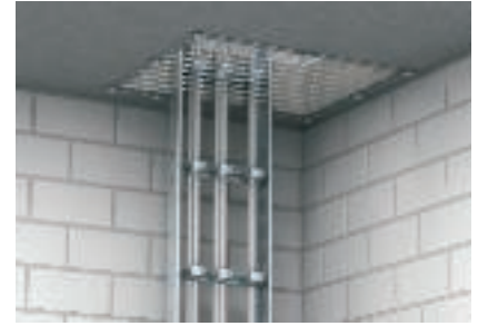
Lock against falling out during ceiling mounting
