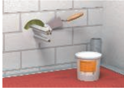
2 cm-deep closure of the surfaces on both sides with the DSX insulation layer creator
