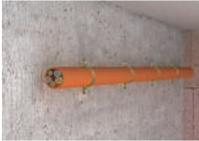
Horizontal cable mounting on the wall
