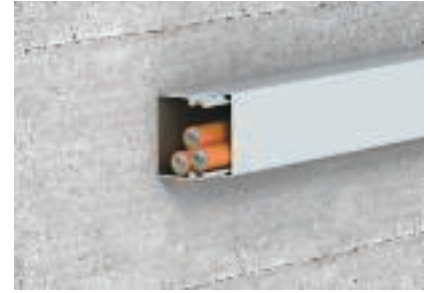
Tidy routing of data and fire alarm cables in the duct, type 20030
