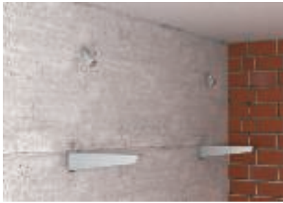
Mounting of the brackets and the connection components on the wall
