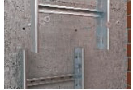
Joint design without connector
