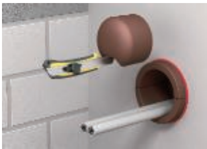
Cutting and mounting of the plugs in the pipe shell
