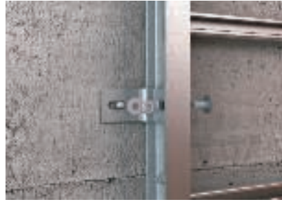
Mounting with screwed-on fastening brackets
