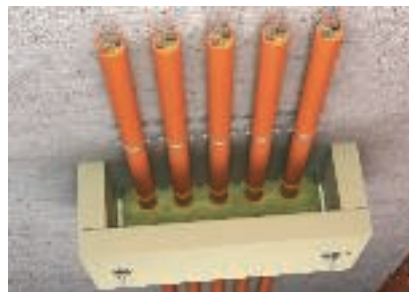
Effective support measure with ZSE90 strain relief
