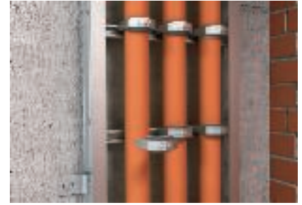
Cable installation with clamp clips on the rungs of the vertical ladder
