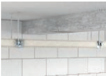
Suspended mounting on the connector elements
