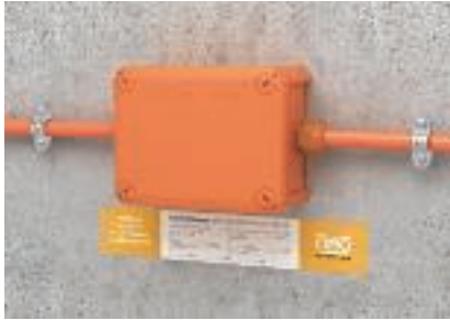
Fully installed FireBox with identification plate
